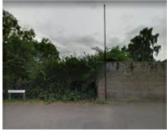
LOCATION 2A WITH POLE
