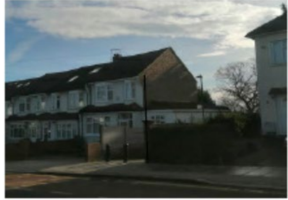
LOCATION 30A WITH POLE
