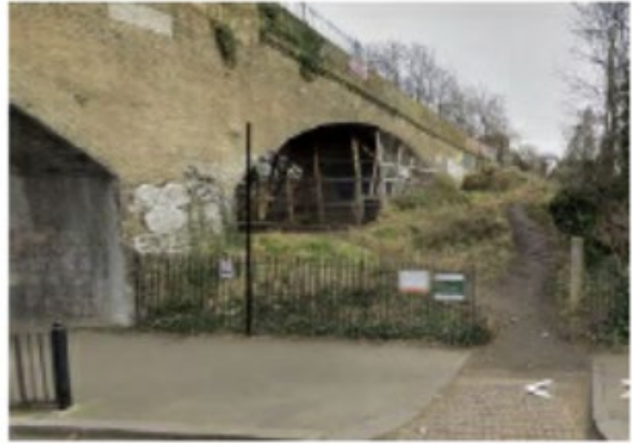
POLE B SOUTH SIDE OF BRIDGE
