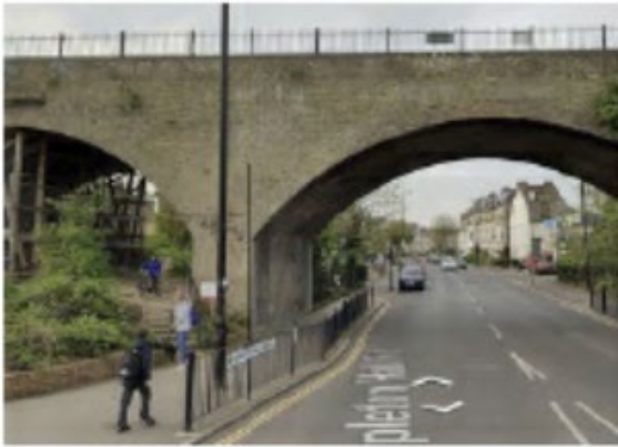
POLE C NORTH SIDE OF BRIDGE
