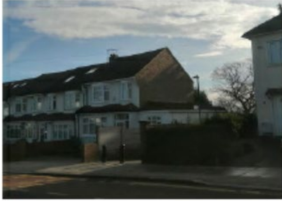
LOCATION 30A WITHOUT POLE
