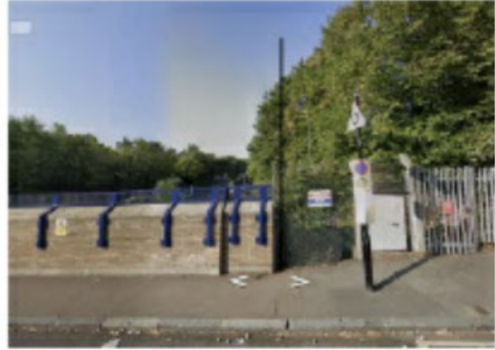
LOCATION 24A WITH POLE
