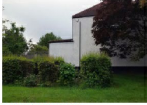
LOCATION 32A WITH POLE
