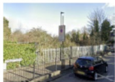
LOCATION WITH POLE + PANEL ON GUARD RAIL
